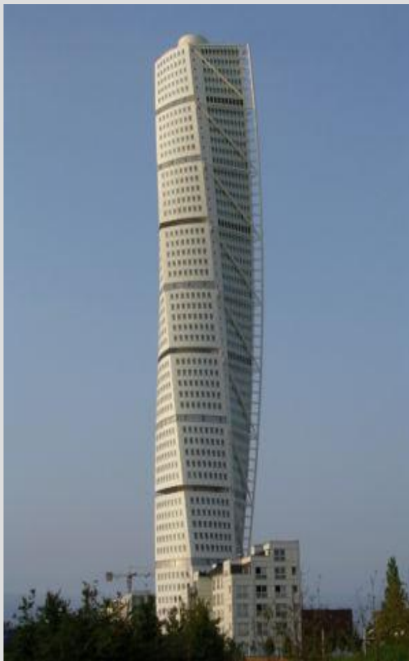
Turning Torso – Malmö, Sweden
