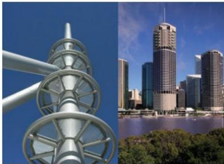
Riparian Building in Brisbane, Queensland (courtesy of Wallbridge & Gilbert)
